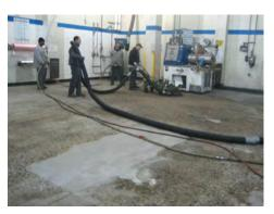
The floor was prepared by total removal of the ½" epoxy topping using 20K water jetting. The floor was left with aggregate show and left damp.
