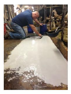
**Description** AGRI -ROK Concrete Overlay is a 1-component, rapid hardening, early strength gaining, cementitious, overlay material for concrete.
