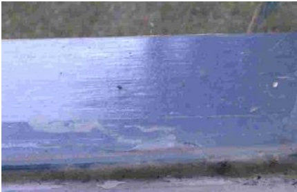
Picture 12: Window Sealant (done while wet)
