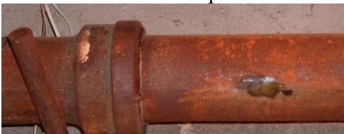
Picture 4: Cast Iron Repair
