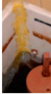
Picture 9: Ceramic Tank Sealant
