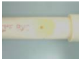
6. Remove NSR Tab. Completed repair. Note resin covers an area larger than the actual hole.
